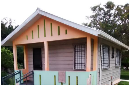
Guest House #1 – Completed
