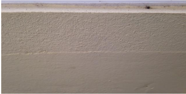
Unfinished walls in dining area downstairs
