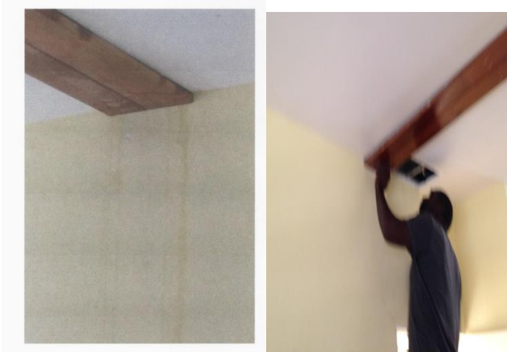
Water - as it came down from the ceiling. Mr. Cruz cut out and repaired section with mold.
